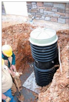
was much less intrusive on Individual grinder pumps installed at each site push our customers and in some slurry of wastewater from homes and other sites to the
